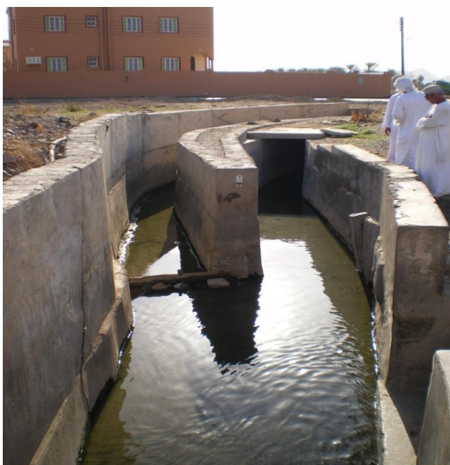
Figure. 5: Low water flow with invention to the canal (wooden piece)
